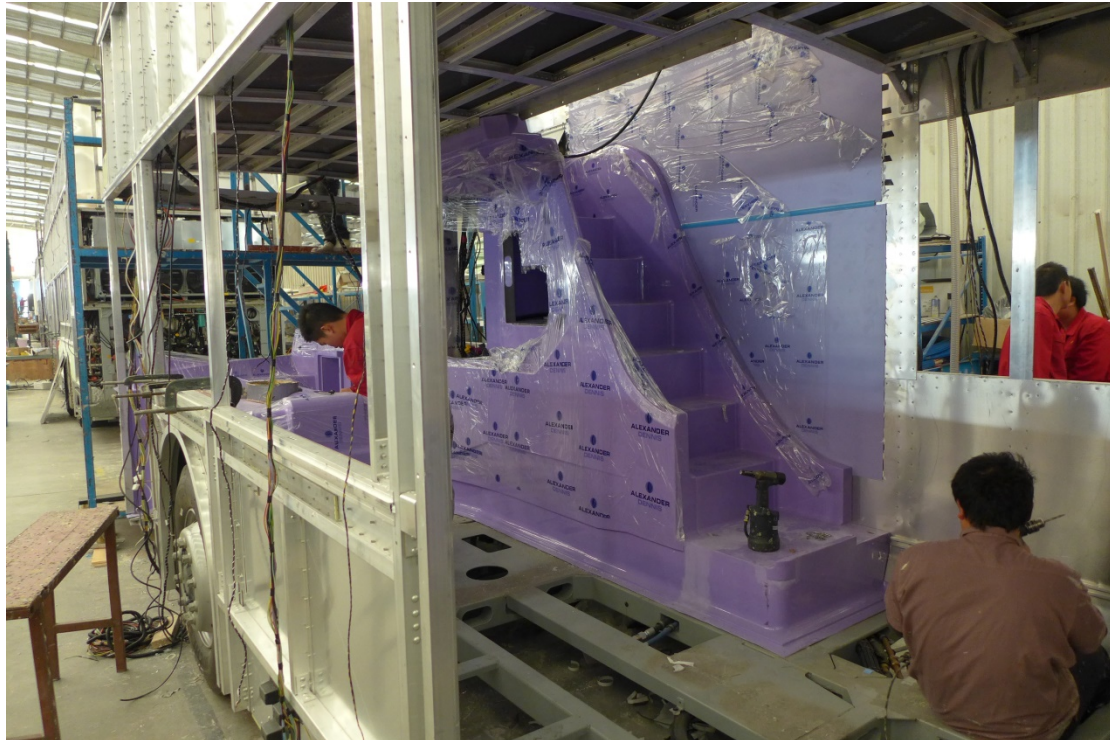
GRP-made ladder module installed in the cabin (Edmund Leung)
